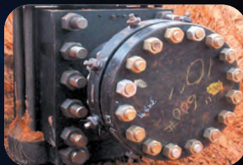
Pipe Repair Services
