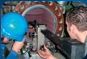
Valve Repair Services
