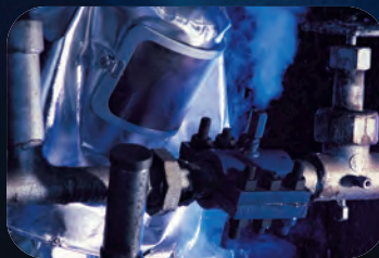
Leak Repair Services
